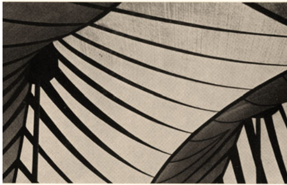
Fig. 1.7 The form of light. Frei Otto, temporary shelter for the Stromeier catalogue, 1954. The covered space is qualified by the designed form of the seams stitching different textile panels, quite evocative of the translucency of natural leaves (Source Morganti 1965)
