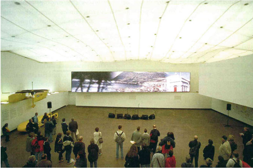
Fig. 3.4 Example of a multi-layer membrane installed into the Portuguese Pavilion, Expo 2000, Hannover, Germany: the number of layers is increased with differing functions (Source Zanelli 2007)
