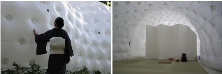
Fig. 1.9 The soft form. Kengo Kuma Architects: Temporary Tea House, made of two textile membranes stabilized by inner air pressure. A perimeter steel U profile connects the two layers of membranes and also works as a temporary foundation (Source Courtesy Form TL Archives)
