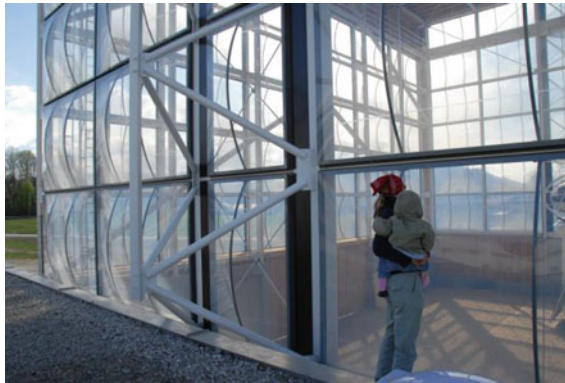
Fig. 4.6 Training Centre for the Bavarian Mountain Rescue in Bad Tölz, Arch. Herzog + Partner (Source Jan Cremers)
