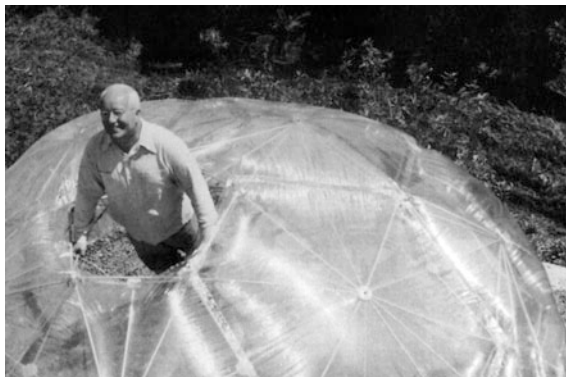
Fig. 1.8 The form of air. Buckminster Fuller, 1949. Transparent pneumatic cushions framed by electrical plastic tubes become a prototype of an ultra-lightweight geodesic dome (Source Baldwin 1996)
