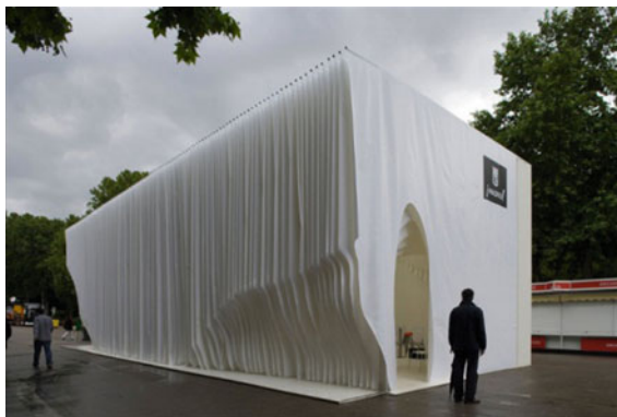
Fig. 1.11 The form of tessellation. Sanina and Marcelo Architects, Madrid, 2009. Following the tessellation concept, an ephemeral house was created by a sequence of textile layers, each one produced in a different manner (Source Courtesy SM Archive)
