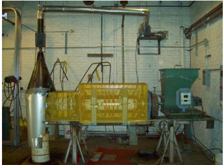
Fig. 17.6 Completed rotary calciner/torrefier at NRRI
