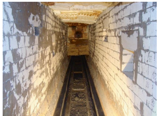
Fig. 17.4 Refractory reline in zones 2–3 of the LHF
