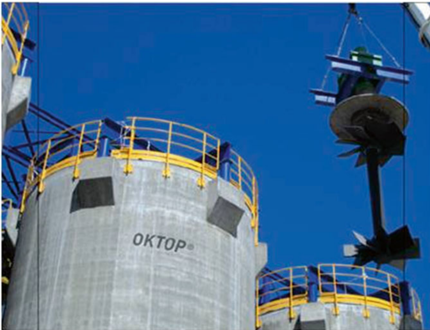
Fig. 12.5 Mixer for agitated tanks. Reproduced with permission from Outotec (USA) Inc.
