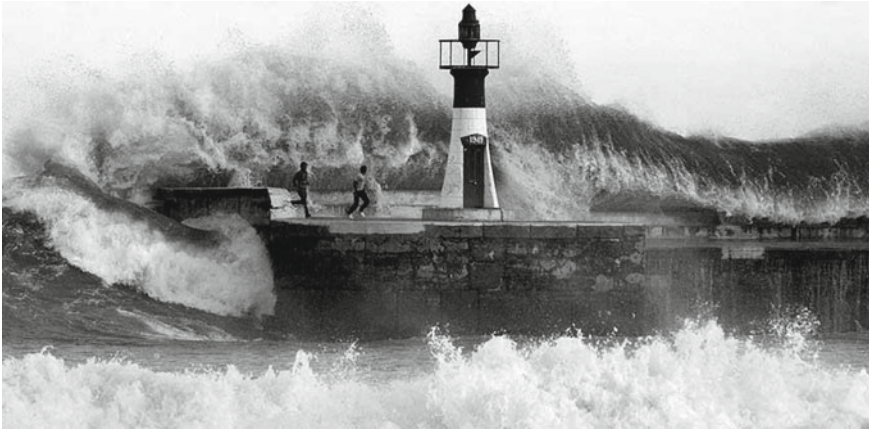
Fig. 1 Freak wave attacks the breakwater in Kalk Bay, South Africa on August 26, 2005
