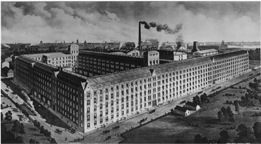
Fig. 15.4 Ericsson's St. Petersburg Plant, 1905
