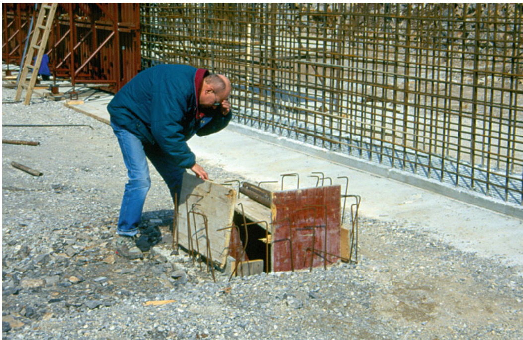
Fig. 1.16 Construction of a road-side artificial entrance
