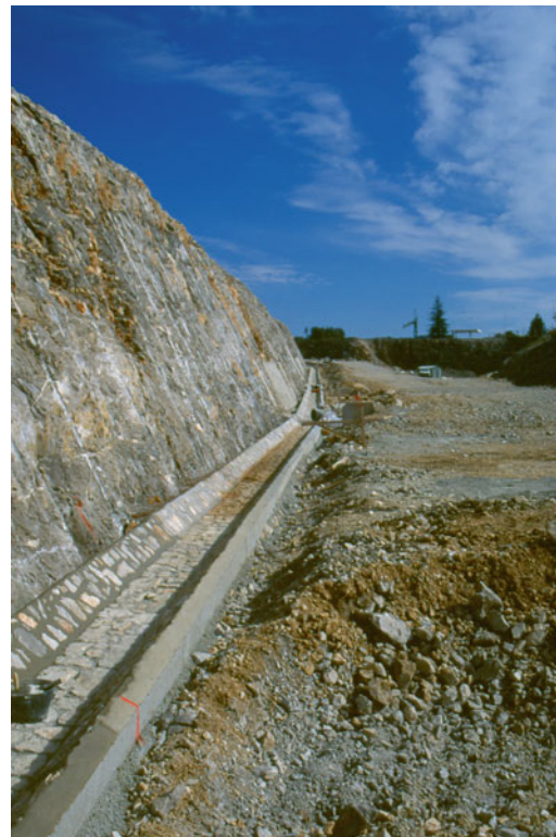
Fig. 1.18 Drainage channels at the side of the road
