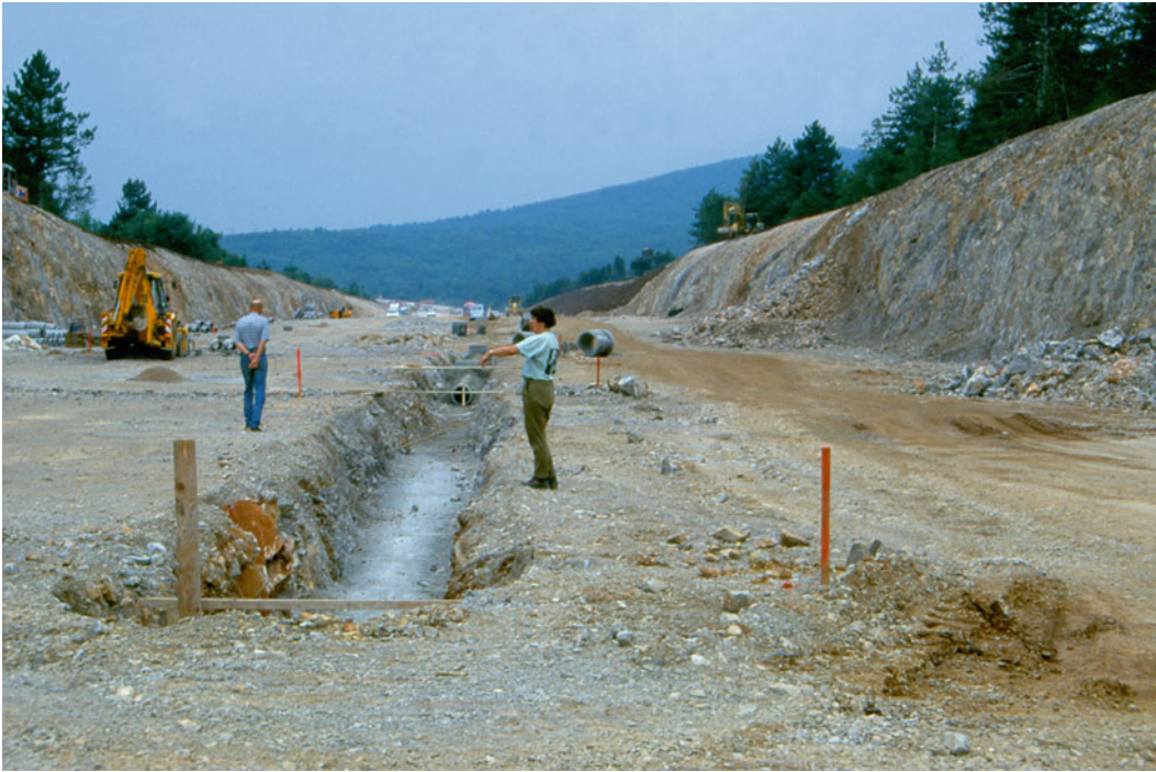
Fig. 1.17 Preparation works for laying pipes for road drainage
