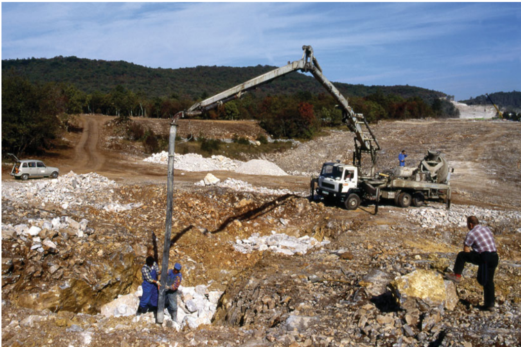
Fig. 1.5 Closing up a fissure cave
