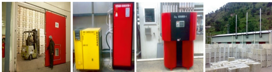
Fig. 9.5 CA storage, N 2 generator, CO 2 scrubber, plastic bins
