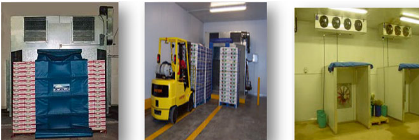
Fig. 7.4 A forced air coolers loaded with boxes ( left ) under loading ( middle ) empty ( right )
