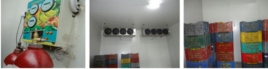
Fig. 7.5 Ethylene cylinder for gassing ( left ), cooling system ( middle ), ripened banana ready for dispatch ( right )
