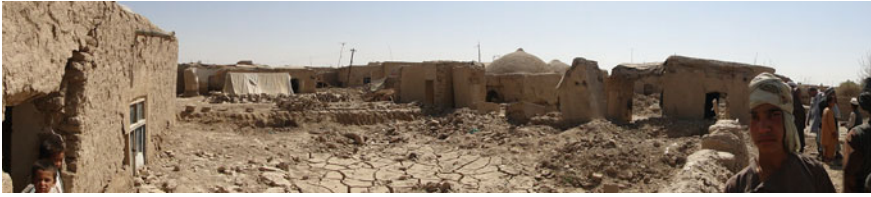
Fig. 2 Flooded houses in Northern Afghanistan. Note the silting up to the window
