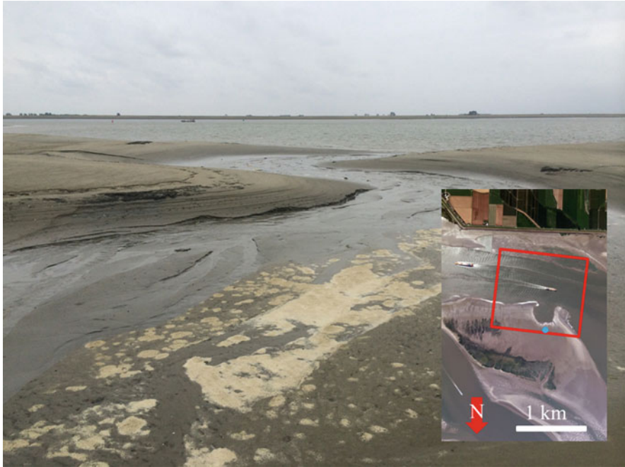
Fig. 24.2 View towards the South from Plaat van Walsoorden sand flat at location of 22 nd of July 2014 flow slide. Inset aerial view. Scar of flow slide clearly visible. Blue dot is position of photo. Test area indicated by red square, see also Figs. 24.1 and 24.3
