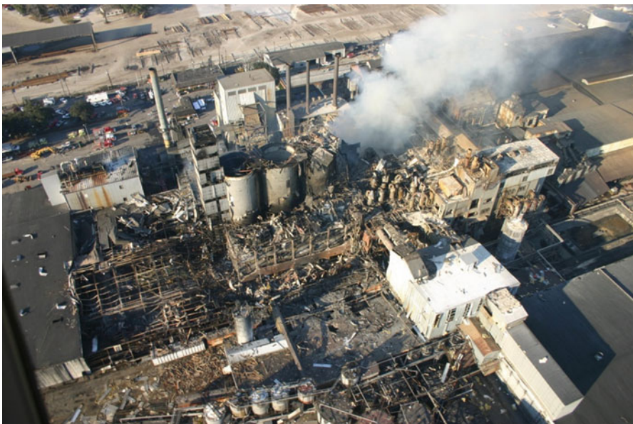
Fig. 14.7 Damaged sugar refinery in Port Wentworth by a dust explosion in 2008 ( www.foodprocessing.com.au )
