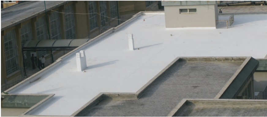
Fig. 20.14 Implementation of a cool roof system in a school in Trapani, Italy
