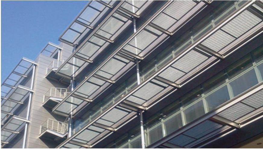
Fig. 21.2 Non-opaque overhangs used for shading. Such systems control solar radiation not only because of their form (overhang) but also due to their steel gratings (flat metal bars)
