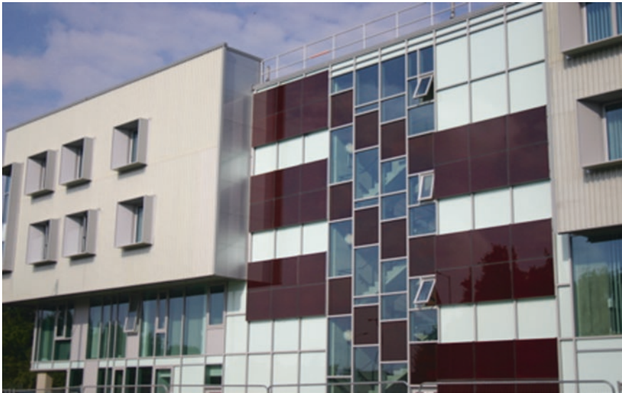
Fig. 18.14 A curtain wall system integrated in the Future Business Center (FBC) in Cambridge ( www.polysolar.co.uk )
