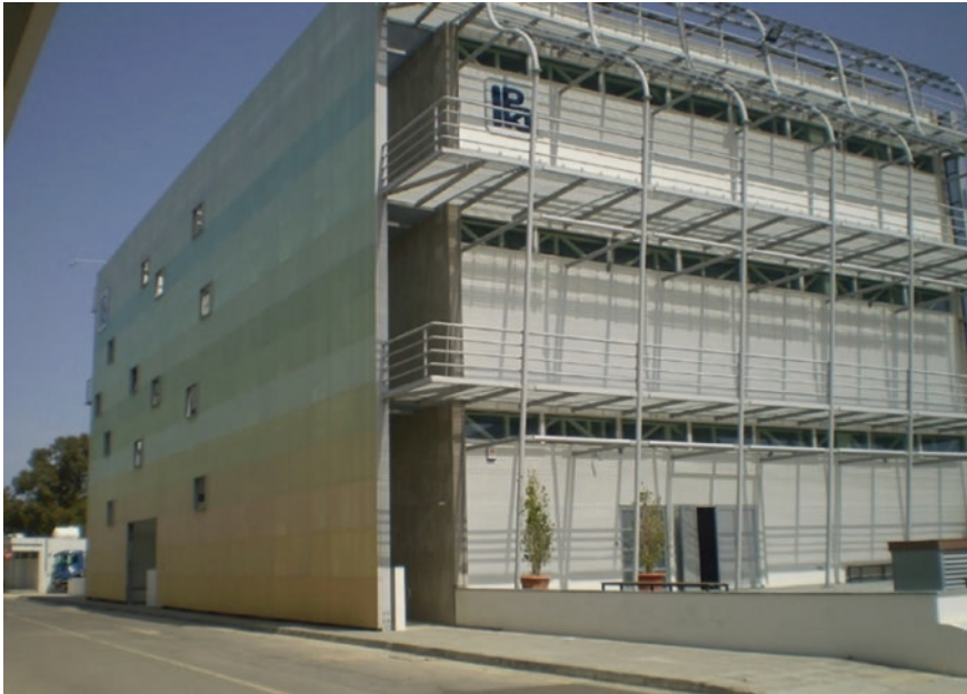
Fig. 10.5 The EEWRC laboratory building
