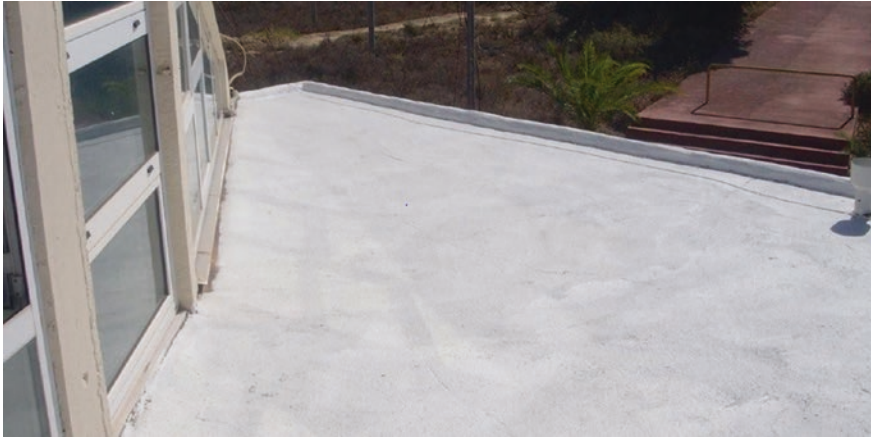
Fig. 20.17 The cool roof installation in Heraklion, Crete
