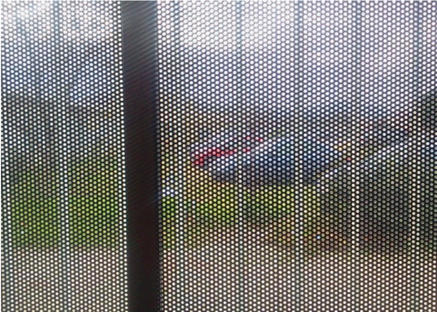
Fig. 21.12 Visual contact with the exterior environment through a perforated metal sheet
