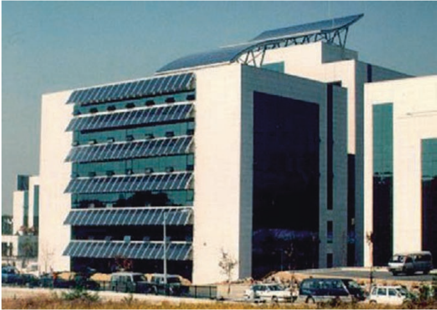
Fig. 18.16 Example of PV for sun screening (PURE project)
