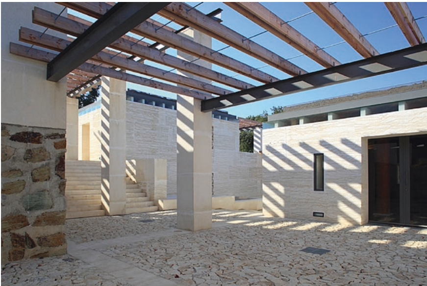
Fig. 24.11 G. Perraudin, Musée du Vin, Patrimoine, Corsica, 2011. View of the outer space and of the massive walls enclosing the buildings
