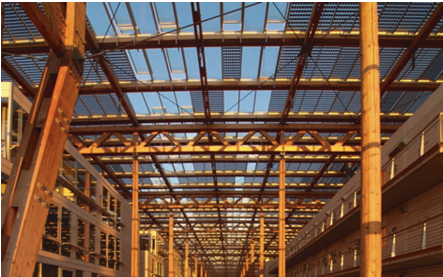
Fig. 18.12 A PV system replacing the roof of the building (commons.wikimedia.org)
