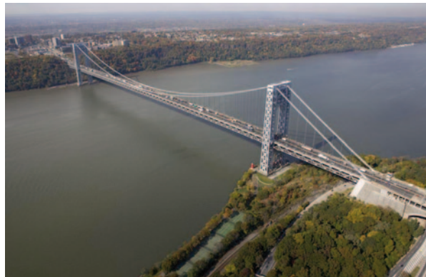
Fig. 2.2 The George Washington Bridge: the long trek from Spanish Harlem to New Jersey
