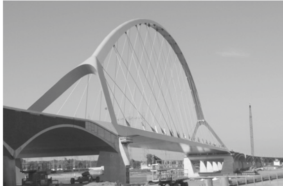
Fig. 1.1 Nijmegen city bridge “De Oversteek” during its construction (September 2013)
