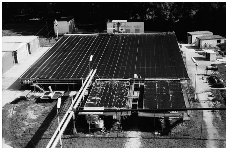
Fig. 5 Outdoor large-scale cascades for cultivation of microalgae (50 and 900 m 2 ) built in the 1960s. One of the first large-scale research facilities for mass microalgae production was located on the campus of the Opatovický mlýn, Institute of Microbiology, Třeboň (mid 1960s). The units had a plain glass surface, with a slope of 3 %, framed by a steel structure. The transverse baffles 3.5 cm high and 15 cm apart were fitted on the surface to create intensive turbulence in the microalgae layer of about 50 mm
