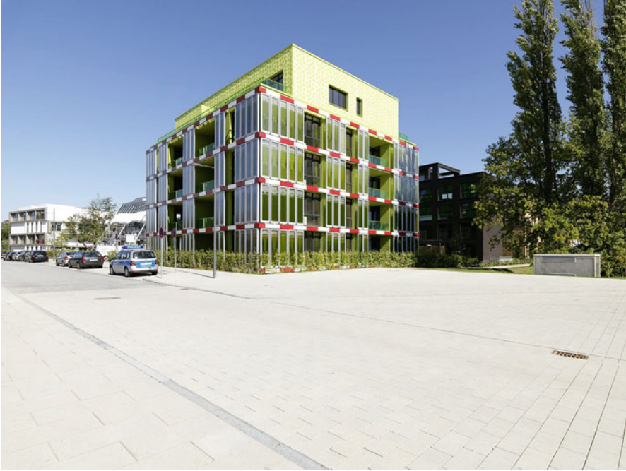
Fig. 23 Photobioreactor façade of the “BIQ-building” in Hamburg (© Paul Ott, Graz, Austria, with permission by Splitterwerk)
