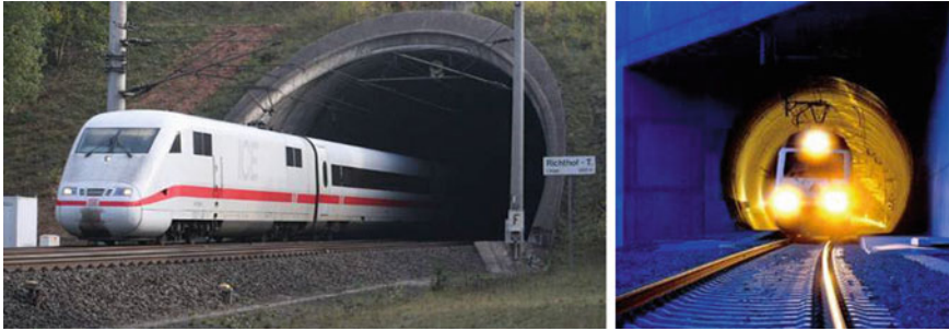
Fig. 6 Portal of tunnel Richtshof of German high-speed rail line Hanover-Wuerzburg and of Loetschberg Base Tunnel; cross-sectional area of tunnels approx. 82 and 45 m 2 , respectively
