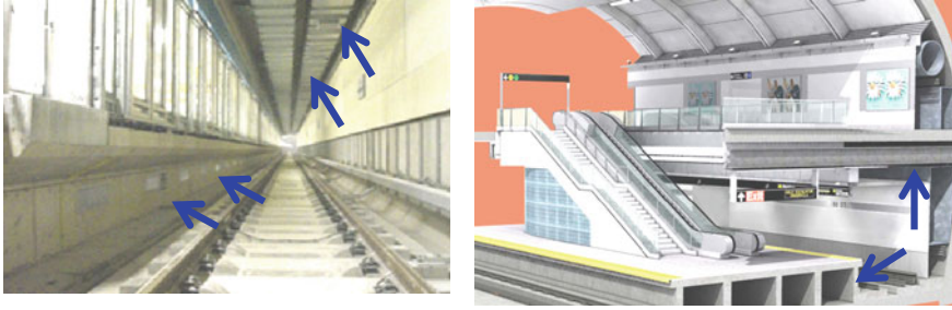
Fig. 9 Heat extraction at station by overtrack exhaust (OTE, top ) and under-platform exhaust (UPE, bottom ) along the station trackway ( left Station trackway along platform, right station model [5])
