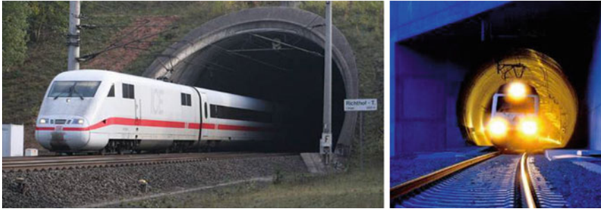
Fig. 6 Portal of tunnel Richthof of German high-speed rail line Hanover-Wuerzburg and of Loetschberg Base Tunnel; cross-sectional area of tunnels approx. 82 and 45 m 2 , respectively
