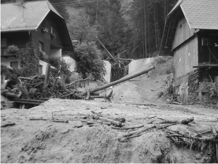
Fig. 3.3 Debris-sorting dam in the “Rauschergraben” (community of Gasen, Austria). Impaired function and overload because of “woody debris”. The measure could avoid heavy losses in the settlement (photograph by WLV Styria, Ellmer)
