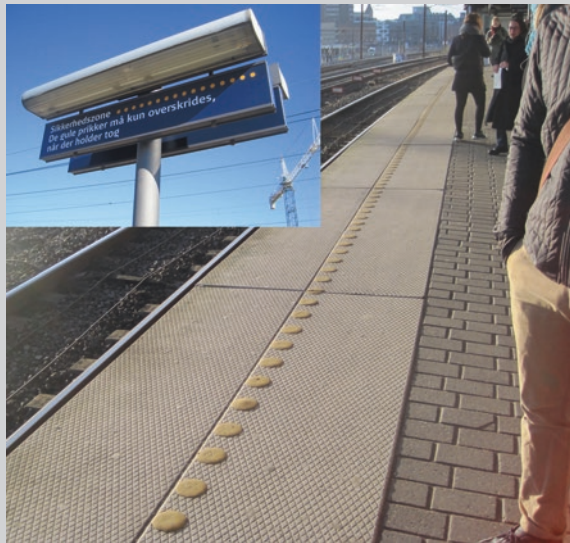
Fig. 11.3 Platform with warning sign (saying: The yellow dots may not be passed if there is no train) and marked risk area
