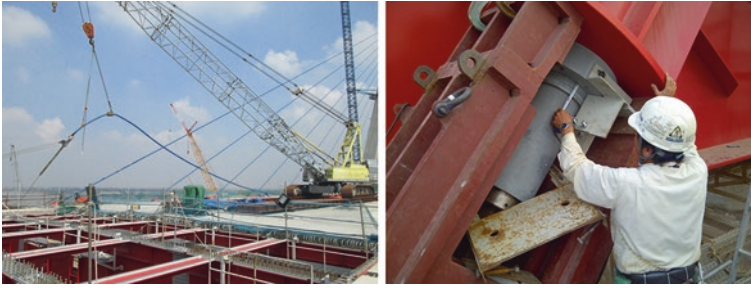
Fig. 15 Installation of stay cable (girder side) and adjusting shim plate
