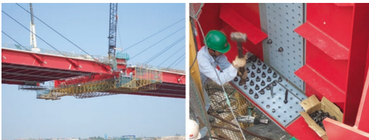
Fig. 17 Installation of closure block and drifting pin to bolt holes
