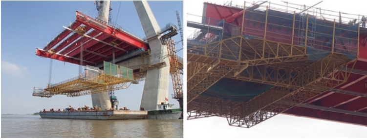
Fig. 11 Lifting up working platform and installation of working platform
