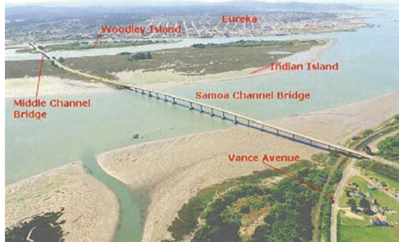
Fig. 1 The Samoa channel bridge
