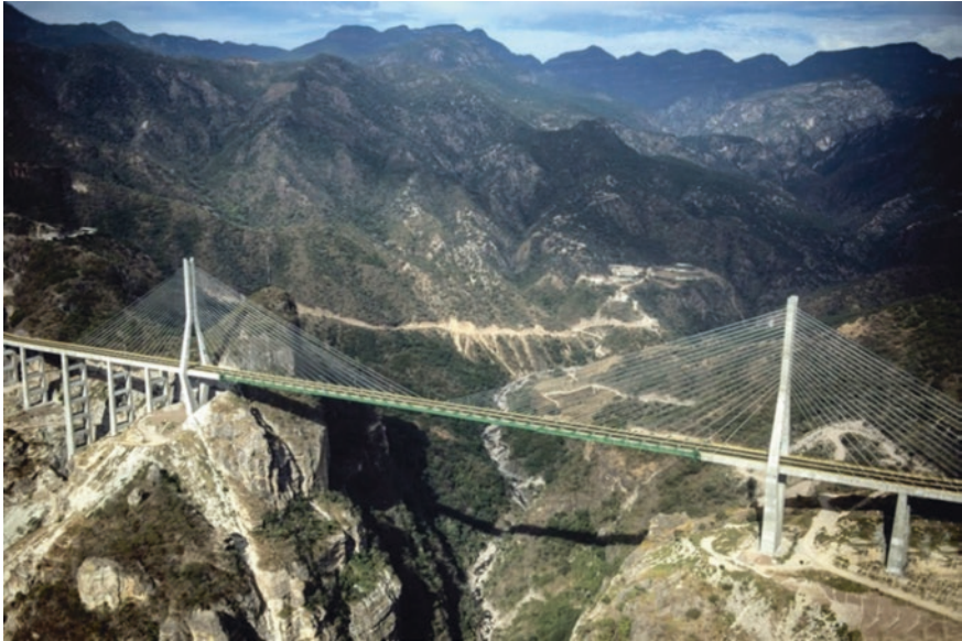
Fig. 1 The "Baluarte" bridge, panoramic view
