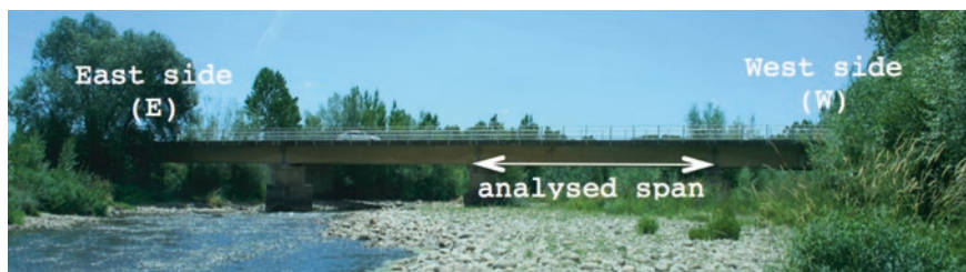
Fig. 1 General view from the North side of the bridge
