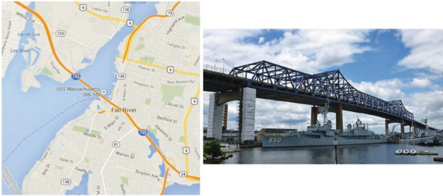
Fig. 1 The location of the bridge on the map, and an image of the north elevation of the bridge [7]
