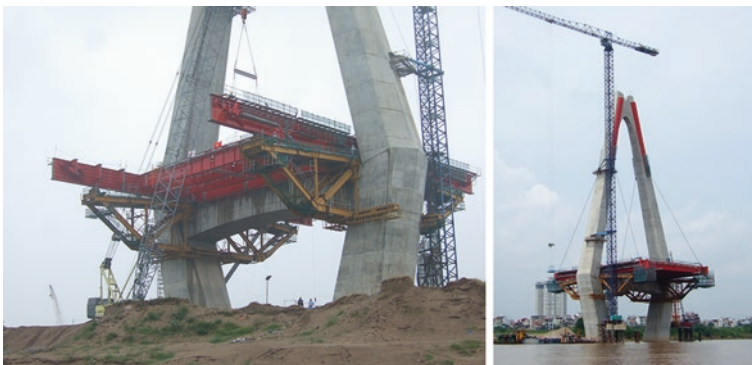
Fig. 7 5 block erection around pylon and Installation of 1st Cable
