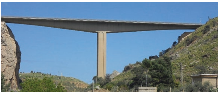
Fig. 8 San Leonardo viaduct in Sicily
