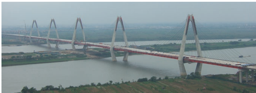
Fig. 1 All view of bridge after closing
