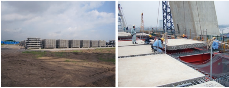
Fig. 13 Pre-cast concrete deck panel stock yard and installation on steel girder
