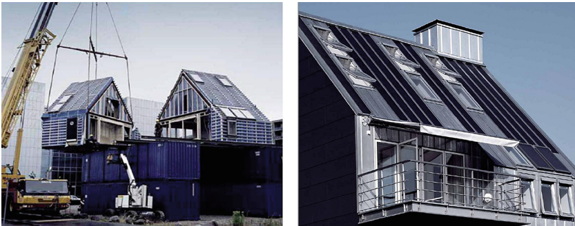
Fig. 2. SOLTAG project - prefabricated system [3]
