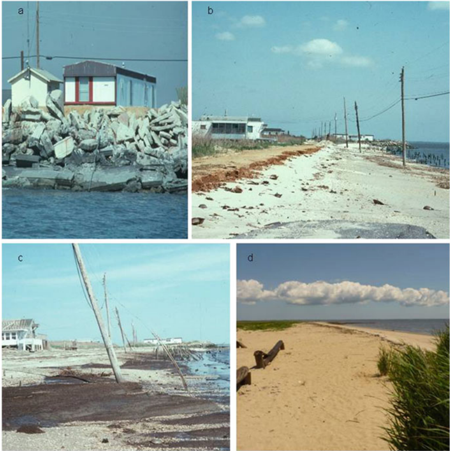
Fig. 3.5 Composite images of Moores Beach, New Jersey showing changes between 1987 and 2014. (a) October 1987, showing the extensive amount of rubble fill used to protect dwellings. The trailer with the red roof seen here is the same as the one in the backgrounds of Fig. 3.5b, c, (b) May 1992, note the pilings in the bay where houses once stood; also note in the foreground a remnant of the older blacktopped road which was washed away, and the reddish colored earthen road to the left which became inundated and impassable, (c) June 1995, the town was essentially abandoned; note the extensive peat formations, a further indicator of beach erosion, (d) July 2014, after the removal of all debris followed by beach nourishment
