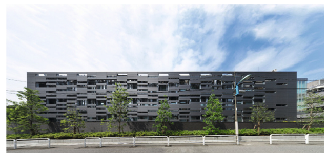
Fig. 1 Front view and Map (upper), and side view (bottom) of TWIns building
