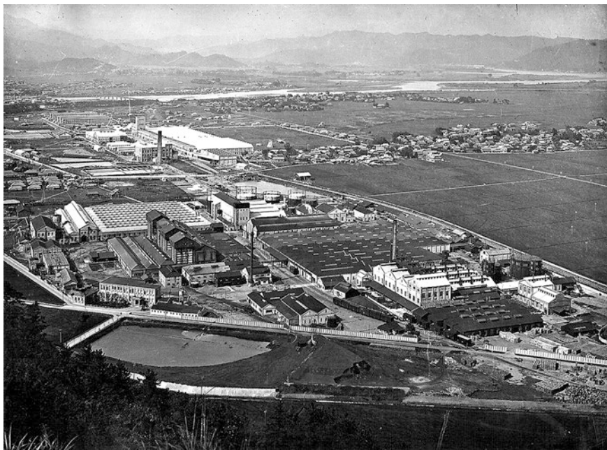
Fig. 5.10 Nobeoka ammonia factory (Casale process), Japan, around 1924. The capacity for ammonia production was 62 tons per day. (Casale SA)
