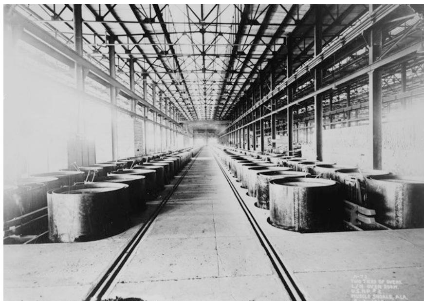
Fig. 5.12 Banks of cyanamide ovens, “U.S. Nitrate Plant No. 2,” Muscle Shoals, Alabama, 2 March 1919. (Library of Congress, Prints and Photographs Division, HAER ALA, 17-MUSHO, 1–65)
