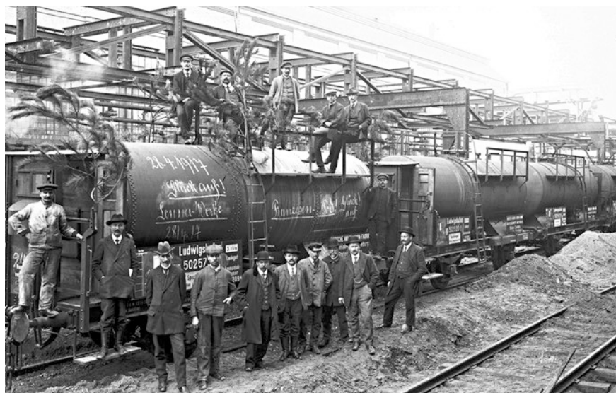
Fig. 4.9 The first trainload of ammonia awaiting departure from the BASF Merseburg works on 28 April 1917, bound for Ludwigshafen, where ammonia was converted into nitric acid and ammonium nitrate. Chalked on the tank of the first wagon are the date, “Good Luck,” and “Death to the French.” Tree branches serve as decoration. (LHSA, MER, 1 525, Fotosammlung, Nr. 786. Landeshauptarchiv Sachsen-Anhalt, Abteilung Merseburg)
