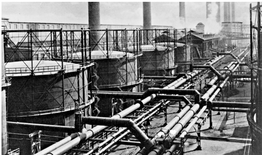
Fig. 4.4 The Merseburg factory, showing the gas plant, with the capacity for producing up to 80 million cubic feet every day. (Bild-Nr XIV/3 Haber, Archiv der Max-Planck-Gesellschaft, Berlin-Dahlem)
