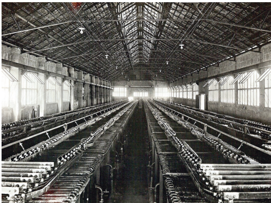
Fig. 5.6 Electrolysis plant for hydrogen used in the Casale ammonia process, at Sabiñángo, Spain. (Casale SA)
