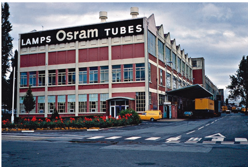
Fig. 2.20 Osram Lamp Division, General Electric Company (from April 1962 Osram (GEC) Ltd), on the GEC North Wembley estate, northwest of London, in the early 1980s. (Osram is derived from Osmium-Wolfram .) From 1923, Robert Le Rossignol worked at the adjacent research laboratories
