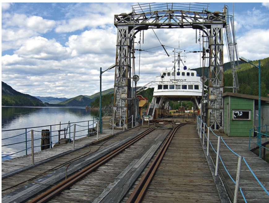
Fig. 2.8 Nitrogen products from Norsk Hydro's remote Rjukan facility were carried by both rail and water transport to the port at Skien, including a railway ferry that plied the 30 km from Mael to Tinnoset across Lake Tinnsjø, and until 1919 a barge from Notodden, on a branch of the Telemark Canal, then on the main canal, to Skien, a distance of 54 km. This is the train ferry terminal at Tinnoset in 2009. (Photo by Nick Lera)
