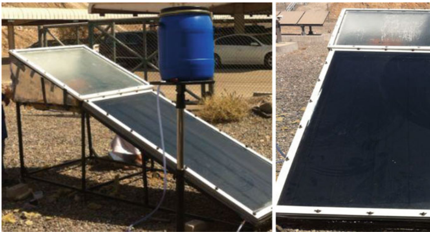
Fig. 3.3 Experimental set up of single slope solar water still with solar energy heating system
