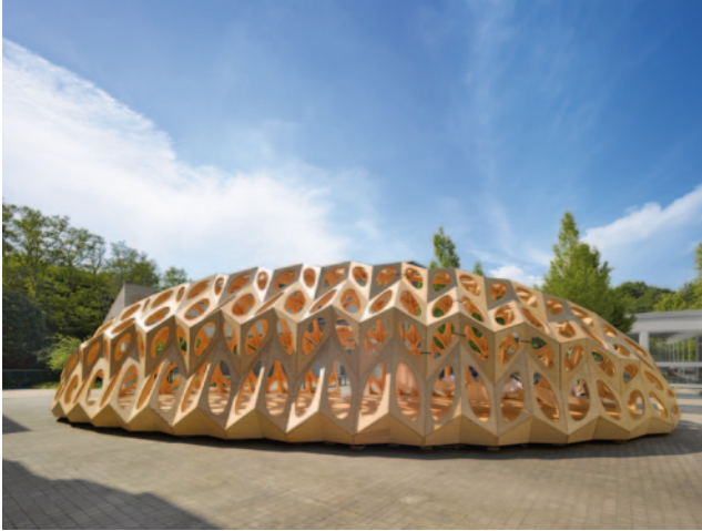
Fig. 6.69 Volume of the BOWOOSS Pavilion amounts to l = 16 m, b = 8 m, and h_{\max} = 4 m
