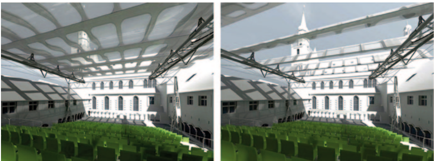
Fig. 6.224 Various open roof positions. The complete retracted position of panels is not represented
