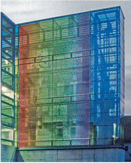
Fig. 6.137 HOE colored facades at the media center of the Bauhaus University Weimar by Pohl Architects
