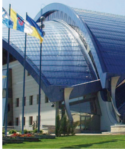
Fig. 6.83 Utilization potential for vaulted sheets: roofing sheet metal for an athletic complex in Odessa, Ukraine
