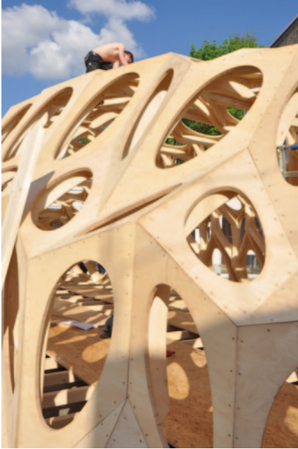
Fig. 6.67 Biomimetic-inspired foldings and hierarchical structuring lead to a perforated envelope. Folding, structure, and opening all guarantee stability. Construction and lighting are integrated members of a materially justified building form
