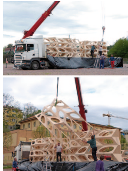
Fig. 6.66 a and b (below) Transporting
