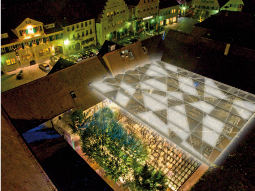
Fig. 6.223 The roof over the monastery courtyard in closed position with light staging
