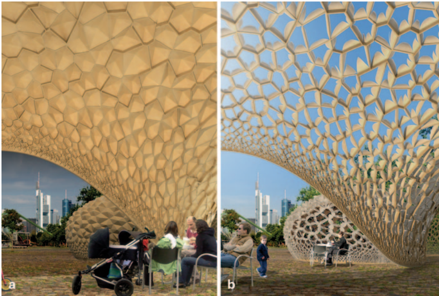
Fig. 6.199 Opening mechanism of a roof structure: left closed (wet conditions) and right opened (dry conditions)
