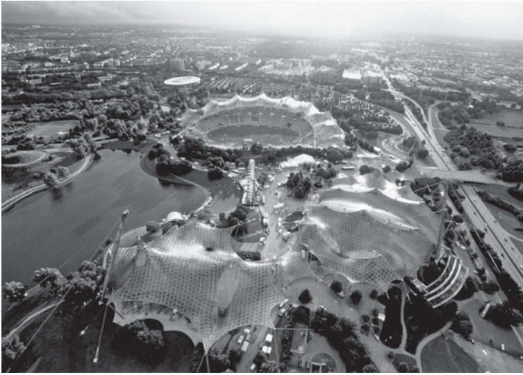
Fig. 3.7 Olympia Stadium in Munich, architects Günther Behnisch and Partner. (Courtesy of G. Pohl)
