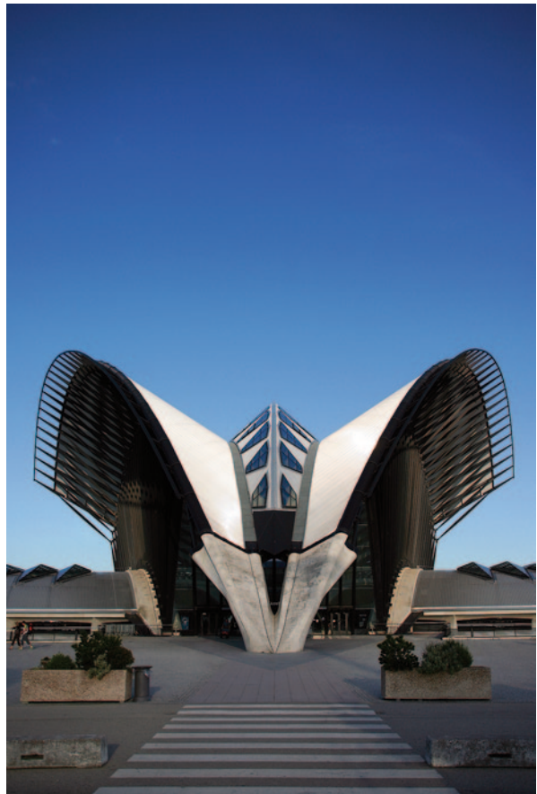
Fig. 3.5 TGV station at Lyon-Satolas, architect Santiago Calatrava. (Courtesy of A. de Luz Mendes)
