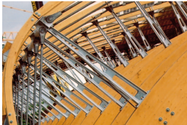
Fig. 3.9 Biomimetically developed, so-called bone struts of the speed skating hall in Erfurt, Pohl Architects. (Courtesy of C. Bansini)
