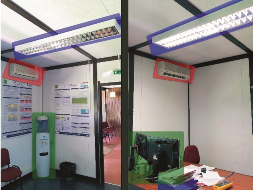
Fig. 1. Monitored loads (blue: illumination; red: HVAC; green: electrical sockets) (Color figure online)
