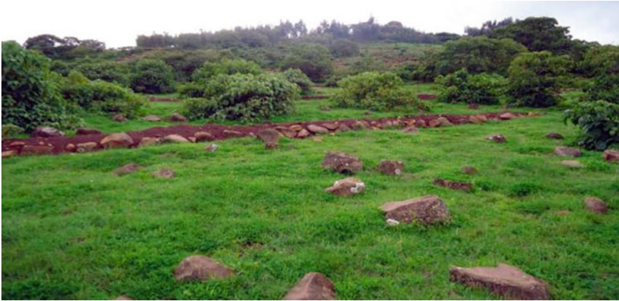
Fig. 35.4 Upper gully treatment measures
