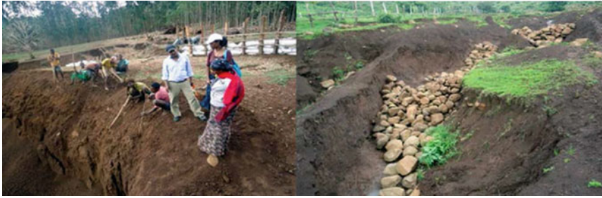
Fig. 35.6 Gully reshaping with steep slope ( left ) and stone use attempt to control gully erosion ( right )
