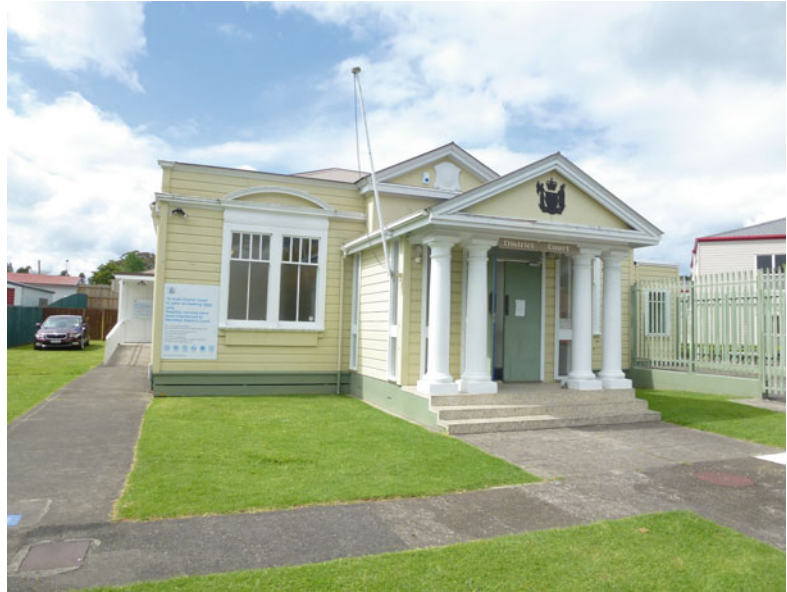
Fig. 8.10 Te Kuiti courthouse, scene of many sly-grogging cases during the era of prohibition in the King Country, and still a functioning Magistrate’s Court today. C.M. King (2013)
