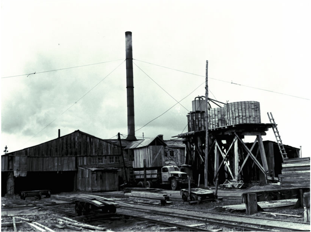
Fig. 5.15 The first mill at Barryville in 1953, built by Marton Sash & Door Co. in 1941. Tramrails lead into the mill from the bush in block A3B2. The truck parked beside the water tower has an MSD sign on the door. This
