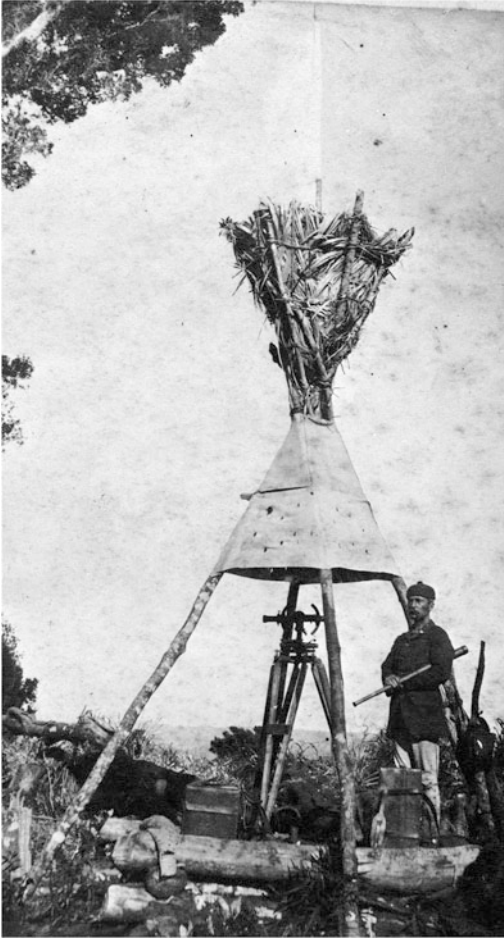
Fig. 5.5 Laurence Cussen with telescope and survey gear at the Maraetua trig point, during the first survey of the King Country in 1883. Hamilton City Library, image 412
