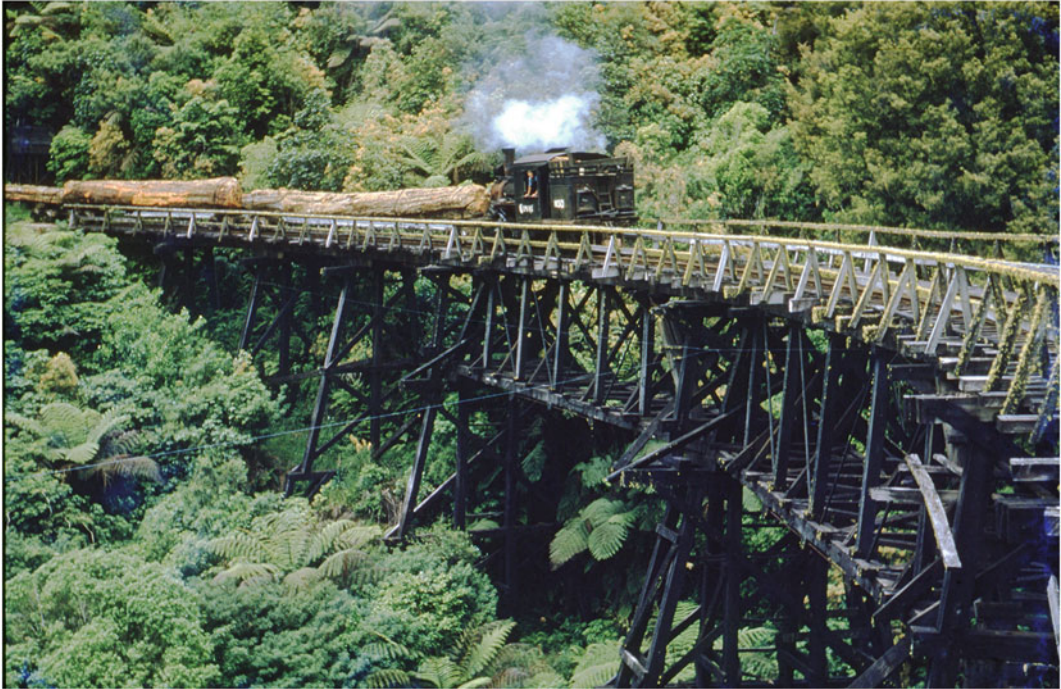
Fig. 5.12 E&B's Climax 1650 lokey cautiously pulling a rake of logs downhill across the Mangatukutuku viaduct towards the mill at Ongarue in 1955. The complex structure of the wooden bridge and the depth of the drop below it are well shown. The engine is running backwards
