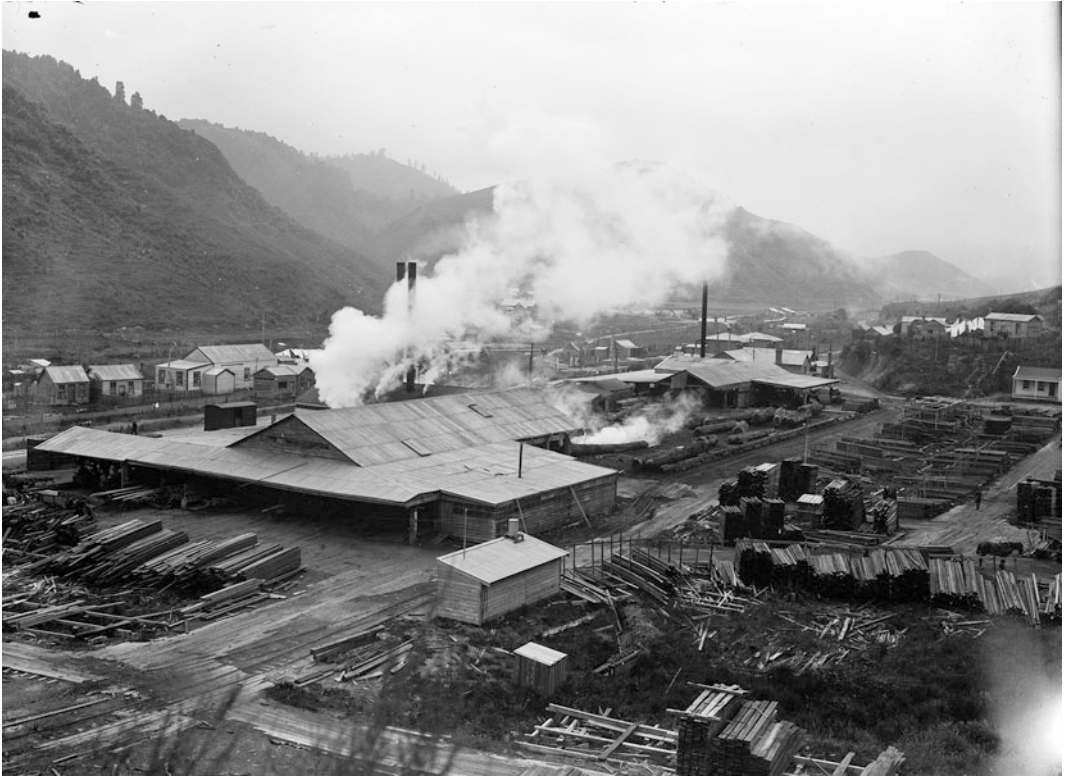
Fig. 5.9 Ellis and Burnand's two timber mills and associated settlement at Mangapehi in 1916. The No. 1 mill built in 1903 ( left ) is wreathed in steam. The smaller No. 2 mill behind it was moved to that site from Tiroa in 1908. Later, two reinforced concrete drying kilns
