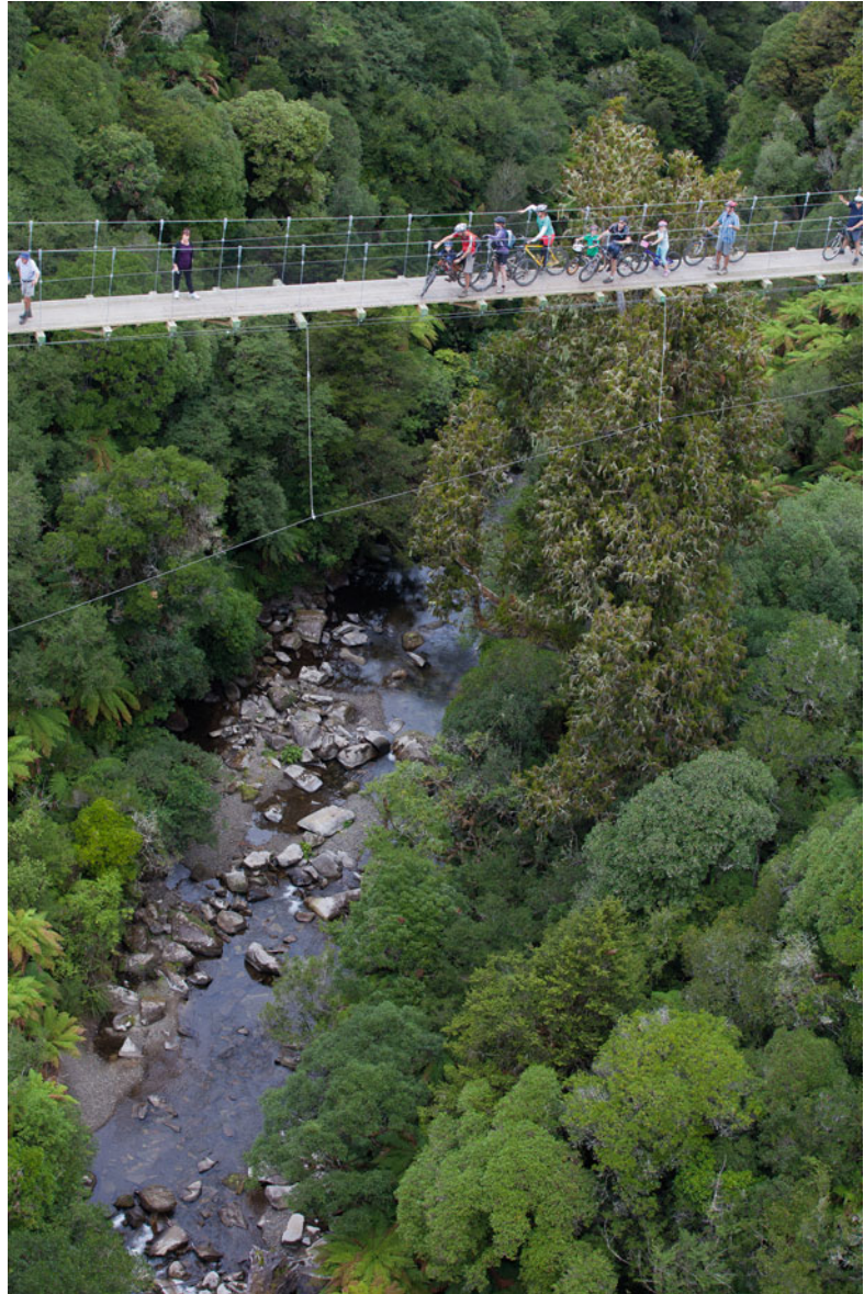
Fig. 14.13 Cyclists on one of the high suspension bridges on the Timber Trail. Marama Shearer
