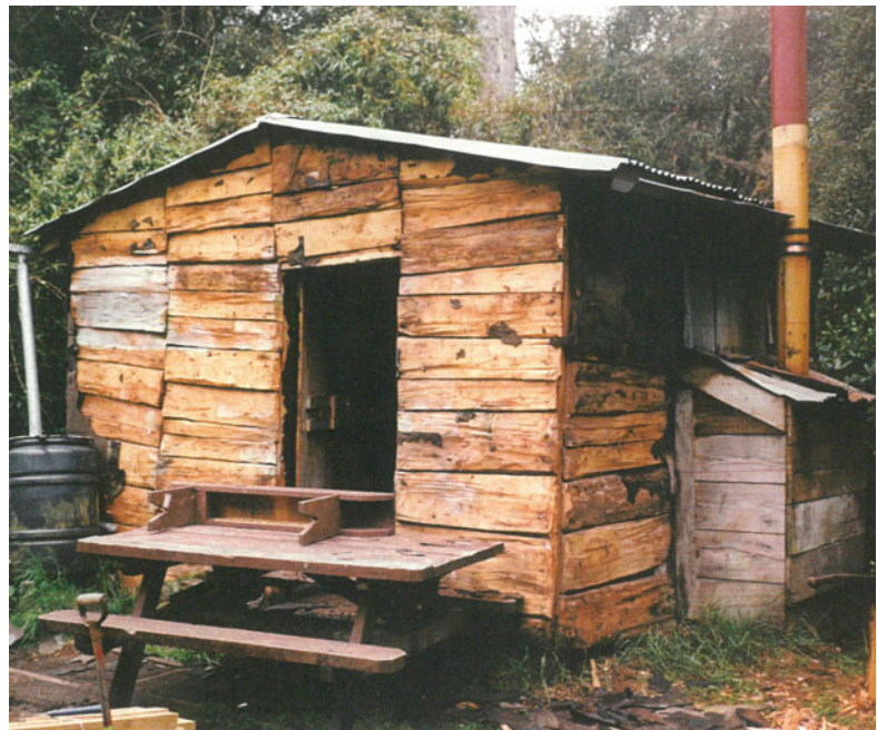
Fig. 14.11 Bog Inn hut was originally built in 1960 close to the Ongarue mire, to support FRI scientists doing research on the forests nearby. NZFS ranger Doug Widdowson was one of the six men who took about ten days to build the hut from split mountain totara planks. Heavy rolls of roofing iron, nails and fittings were air-dropped to the site, but had to be dug out of the adjacent swamp, hence the name "Bog Inn". The hut has been upgraded, and is still a popular destination for trampers. Crown Copyright, Department of Conservation Te Papa Atawhai (1990). Photographer: John Mason
