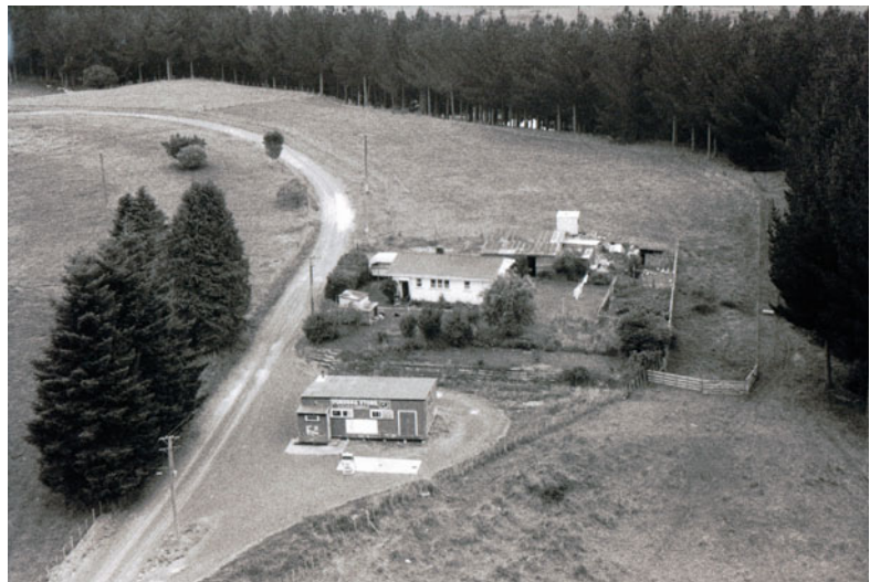
Fig. 8.9 Pureora General Store, and the Russells’ house. Crown Copyright, Department of Conservation Te Papa Atawhai. Photographer: John Mason
