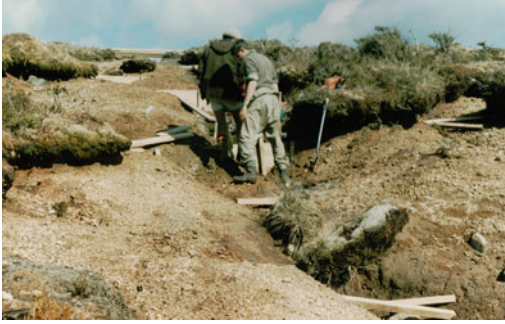
Fig. 1.10 Track repairs on Pureora summit. The pumice deposits covering the peak up to about 1 m deep are soft Taupo ignimbrite erupted c. AD 232. The very high energy release of the eruption enabled the ground-hugging, ignimbrite-generating pyroclastic flow to ascend > 1000 m to overtop Pureora (see Box 1.1). The weakly weathered loose pumice, once exposed and lacking vegetation cover, is very vulnerable to erosion by heavy rain and human traffic. Crown Copyright, Department of Conservation Te Papa Atawhai. Photographer: John Mason
