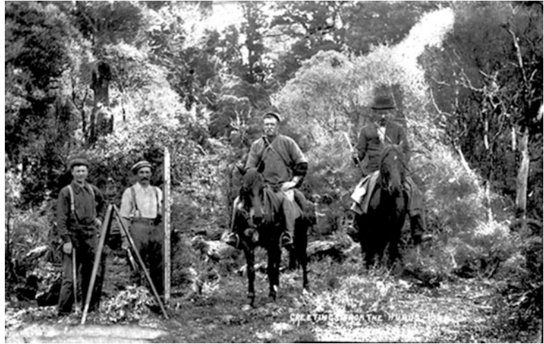
Fig. 5.7 Survey party in the bush, selecting a route for a tramway for the Ellis and Burnand sawmill. Undated, probably early 1900s. Hamilton City Library, image 11641
