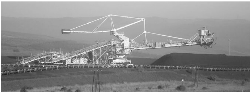
Fig. 7 Area of homogenizing disposal site of Tušimice power plant
