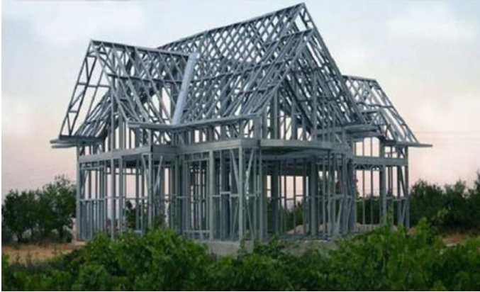
Fig. 1 Steel building of cold-formed thin-walled open sections
