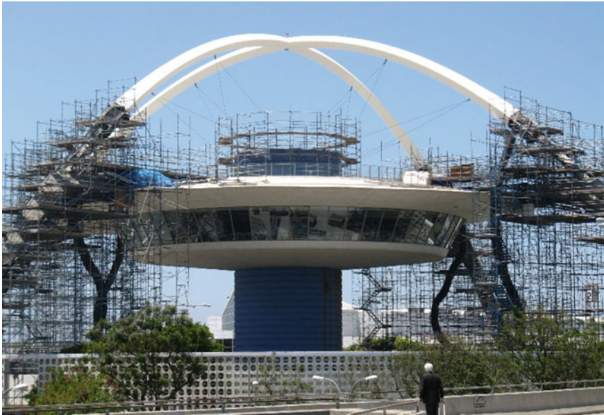
Fig. 2 Theme building in Los Angeles under renovation for seismic retrofit [3]
