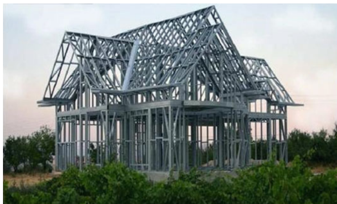
Fig. 1 Steel building of cold-formed thin-walled open sections
