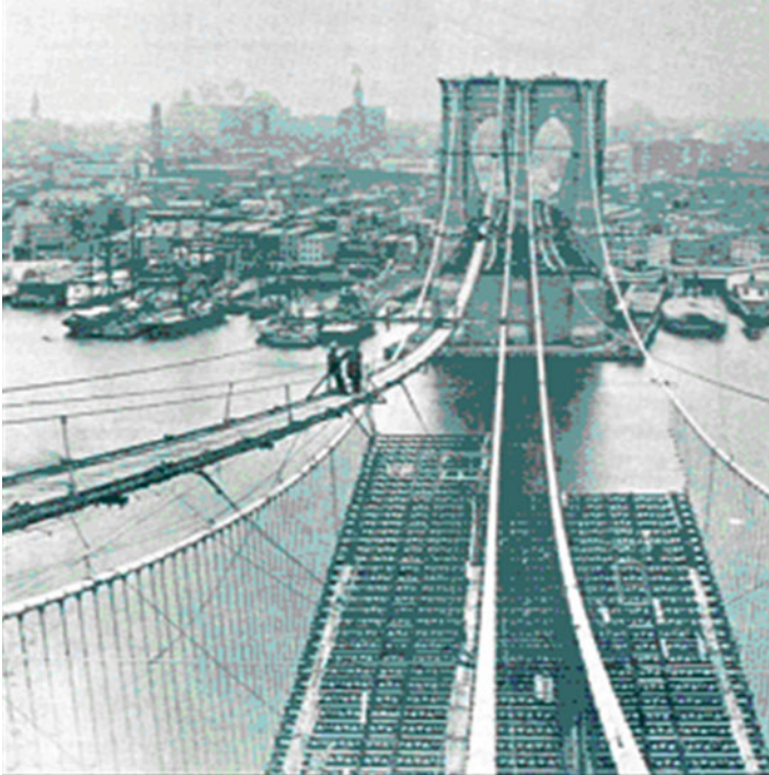
Fig. 50.6 Construction of the Brooklyn Bridge (Source: Museum of New York)
