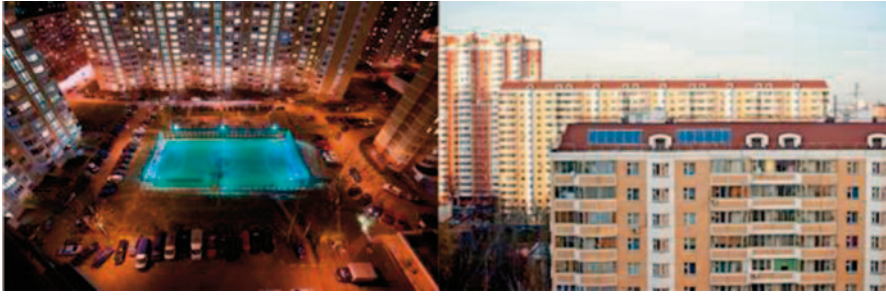
Fig. 20.2 View of the lighting system installed on a sports ground in Moscow (2011)
