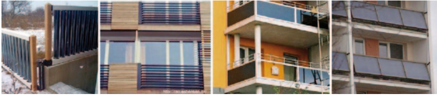
Fig. 64.7 Building-integrated solar thermal system (BISTS) balustrade/railing feature
