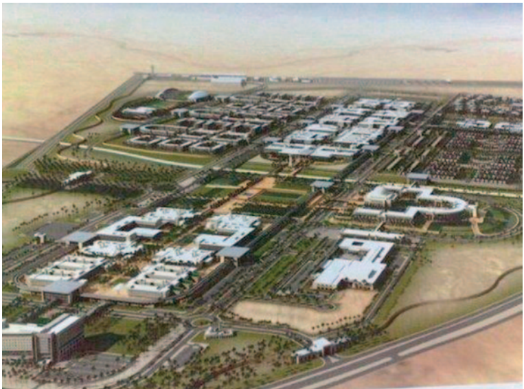
Fig. 28.9 Saudi Arabia's solar thermal plant
