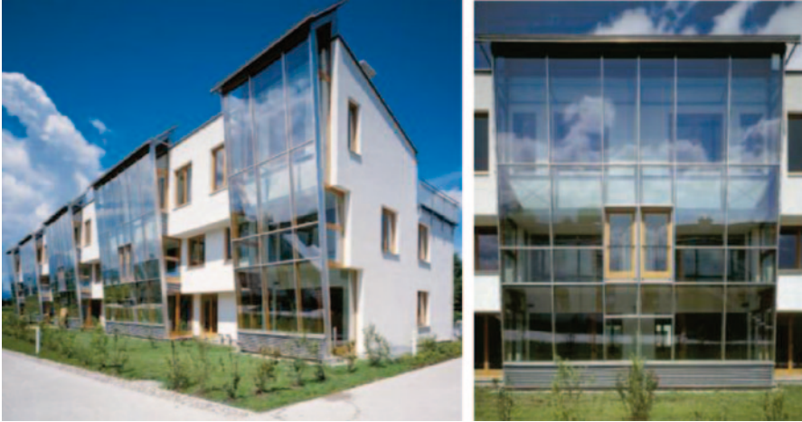
Fig. 83.1 Southern view of the building of Gneiss Moss III, Salzburg, and a view of one of the greenhouses of the building III. (Source: Malighetti Laura, “Una serra in facciata”, in Il Sole 24 Ore—Arketipo , no. 5, 2006)
