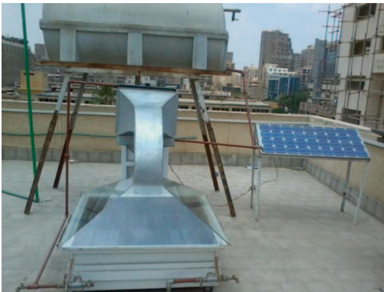
Fig. 75.1 Photographical view of the novel solar industrial wastewater treatment plant
