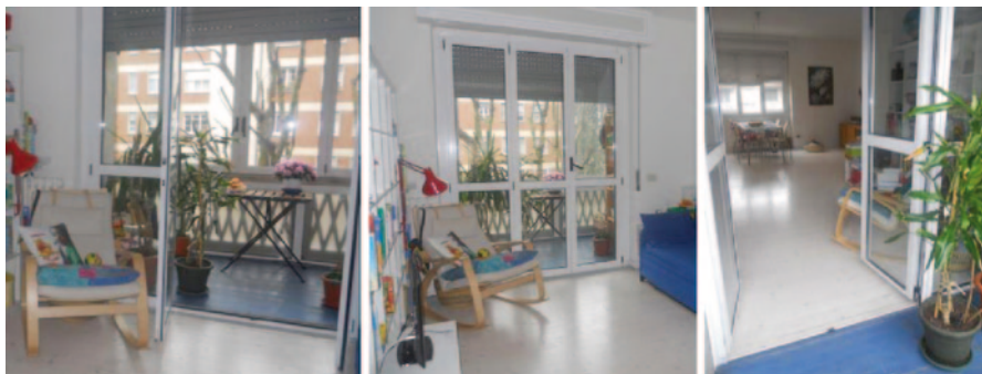
Fig. 83.5 View from inside the solar greenhouse in winter season (closed loggia) with deciduous trees that allow the solar radiation access ( left ). View from inside with the closed French window between the heated space and the greenhouse ( central photograph ). View from the greenhouse to the house ( right )
