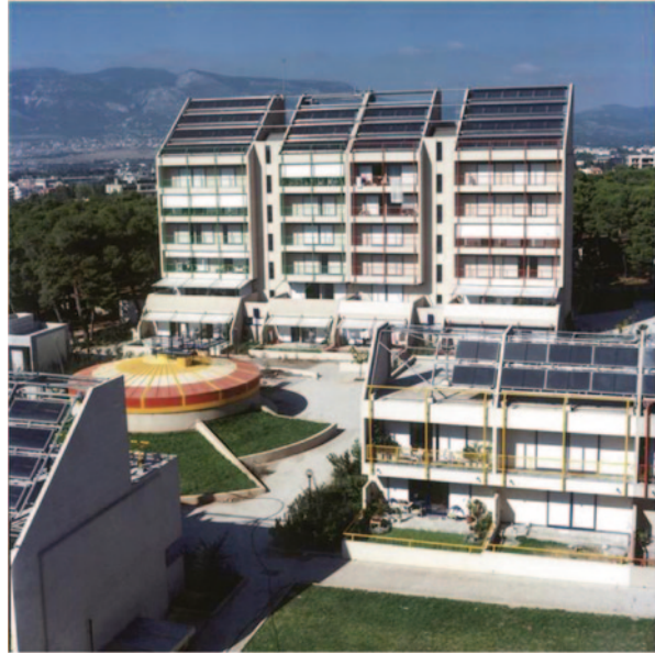
Fig. 72.6 Partial view of Solar Village 3 with the interseasonal storage tank in the front
