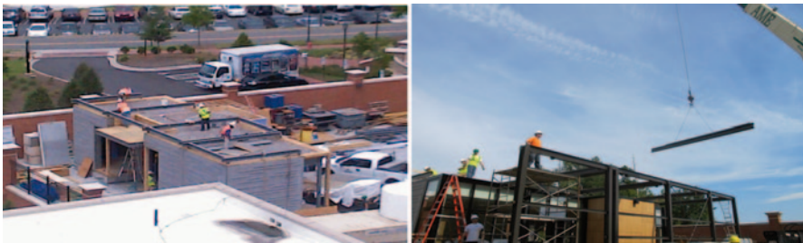
Fig. 61.7 Construction on campus
