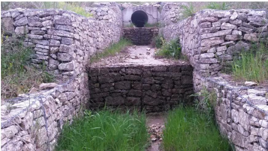
Fig. 4.5 Picture of a stepped gabion weir built in Ripalimosani, Molise (Italy)
