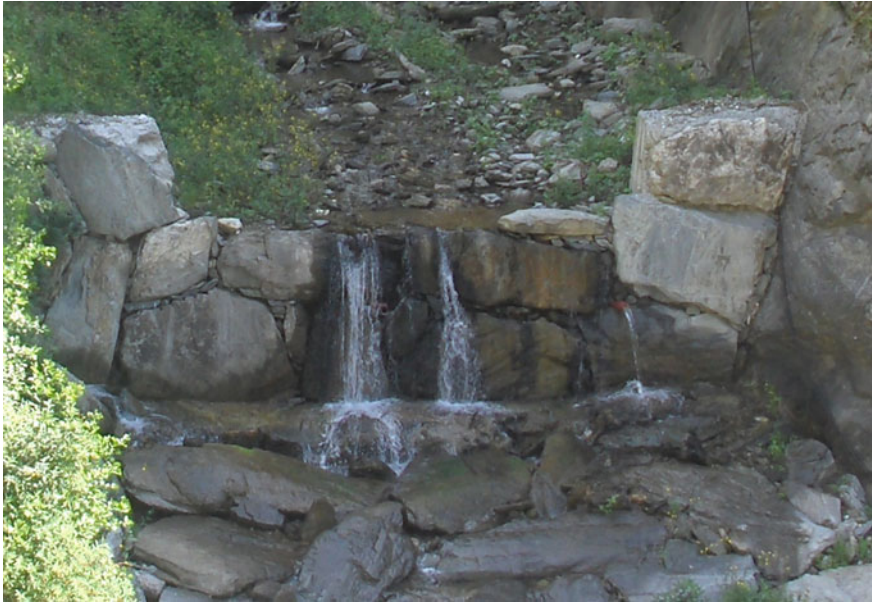
Fig. 4.7 Picture of a rock grade control structure built in Cardoso river (Tuscany, Italy)
