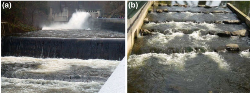
Fig. 9.4 Aeration at hydraulic structures. a Aeration at a weir downstream of Oker dam in Germany; note the strong aeration at the bottom outlet in the background. b Aeration on a cross-bar block ramp due to local hydraulic jumps (Oertel and Bung 2012)
