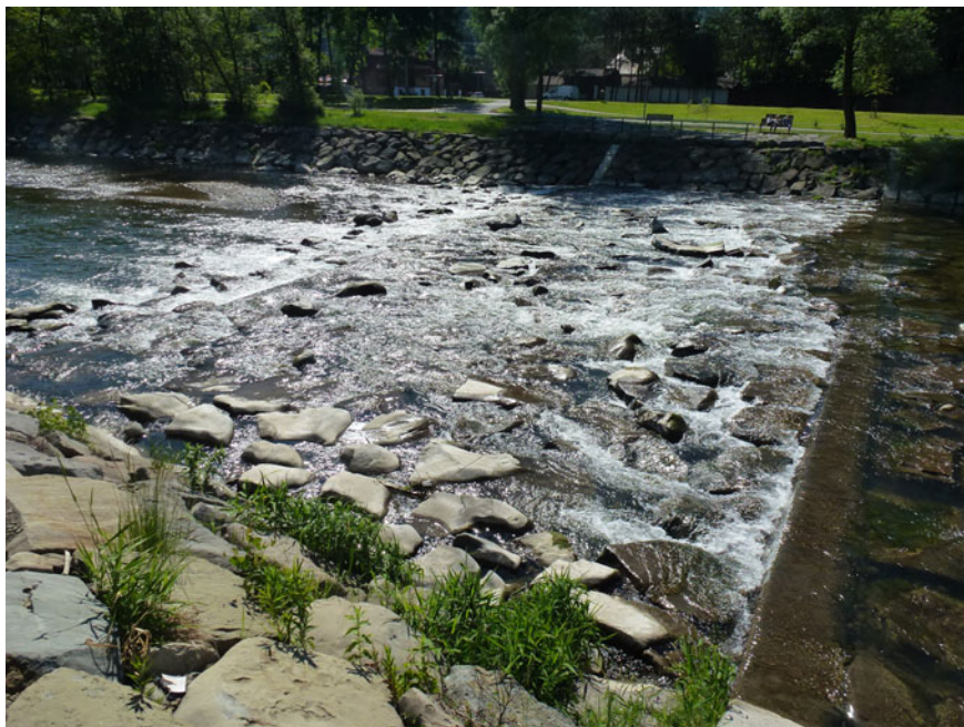
Fig. 4.1 Picture of a block ramp built in a river in the Carpathian mountains (Poland)
