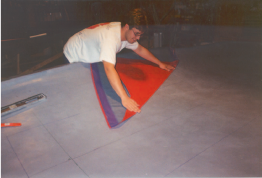
Fig. 11.17 Laying down outer peel ply. (Brian Lisiecki)
