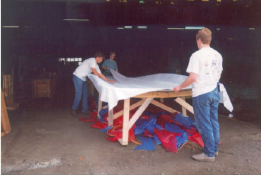
Fig. 11.18 Laying down bleeder cloth. (Brian Lisiecki)
