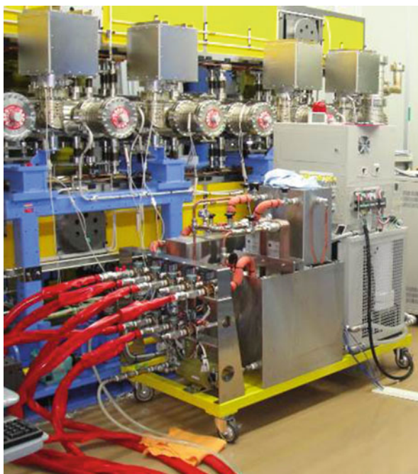
Fig. 18.3 Circulating pressurized hot-water machine for cooling or heating the magnet arrays
