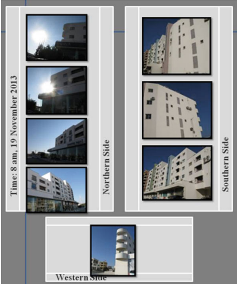
Fig. 28.13 Photos, Mesan Apartment, at 8:00 a.m. (taken by author)
