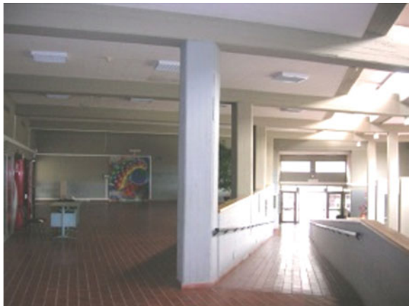
Photo 6 Internal view of the upper atrium
