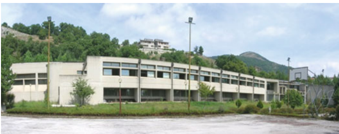
Photo 1 View of South elevation
