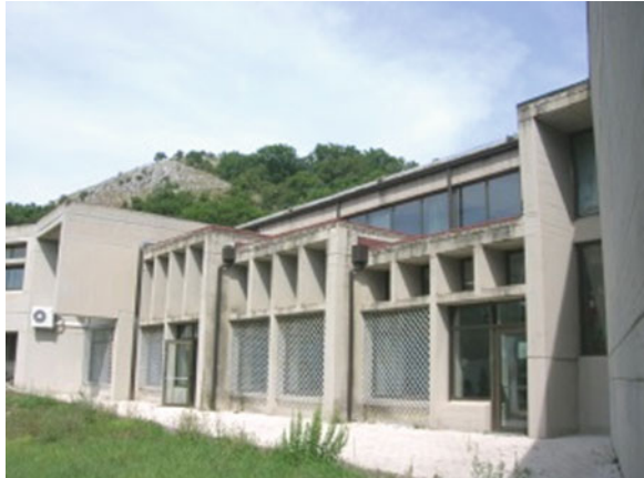
Photo 4 Exterior view of the atrium-library
