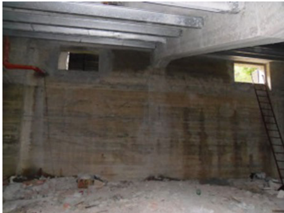
Photo 9 Slab propped up with steel beams
