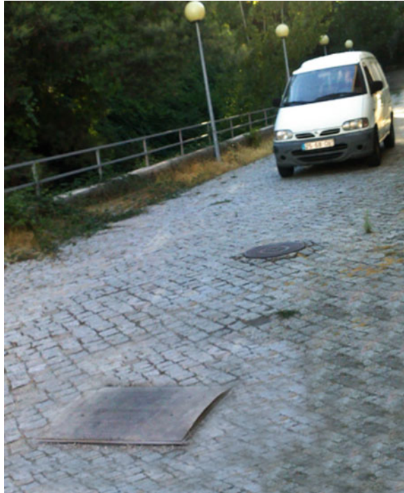
Fig. 1 Waynergy vehicles prototype installed in an access road pavement
