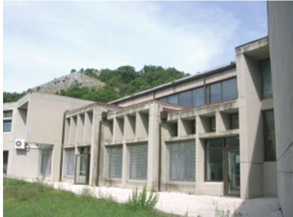
Photo 4 Exterior view of the atrium-library
