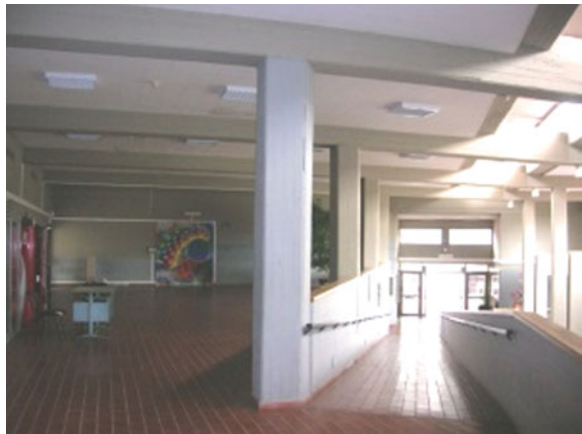
Photo 6 Internal view of the upper atrium
