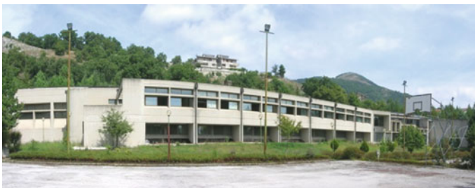
Photo 1 View of South elevation
