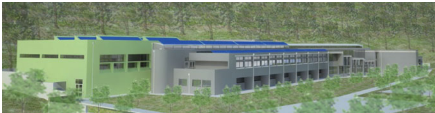
Fig. 4 Overall external view South-East side shows the different color finishes of the main building envelope and Gym, and the placement of photovoltaic panels on the roof of the sheds
