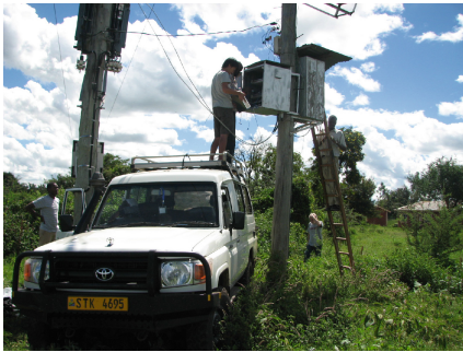
(a) Replacing the Router
