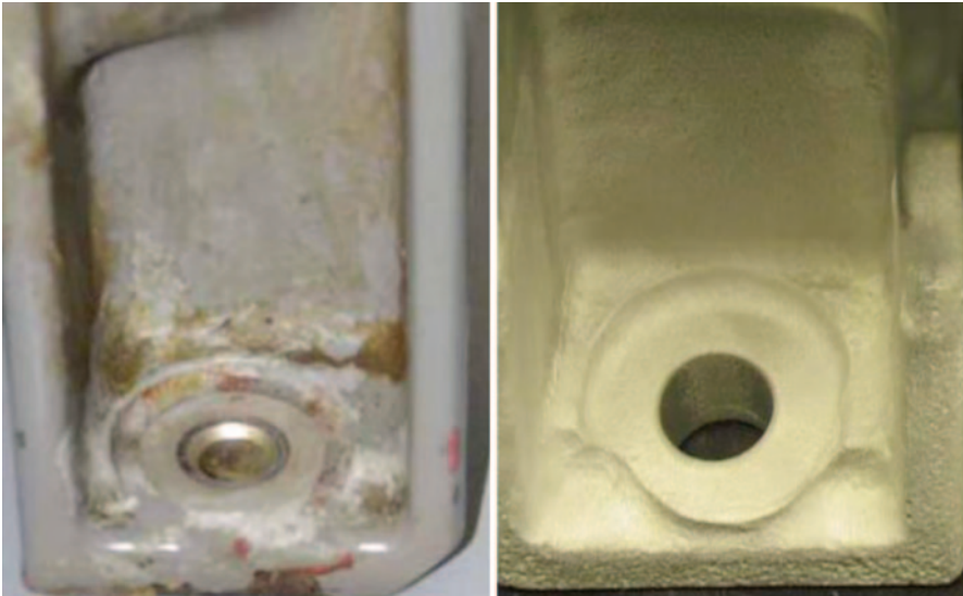
Fig. 10.4 Before and after photos of cold-sprayed restored UH-60 main rotor transmission housing. (Champagne and Barnett 2012)
