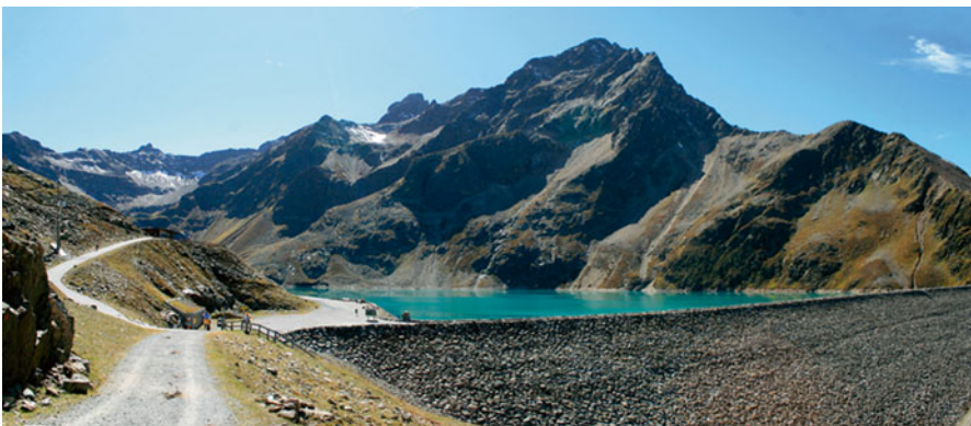
Fig. 6.4 The “Finstertal” reservoir in the K uhntal/Tyrol (Photo Markus Weber)
