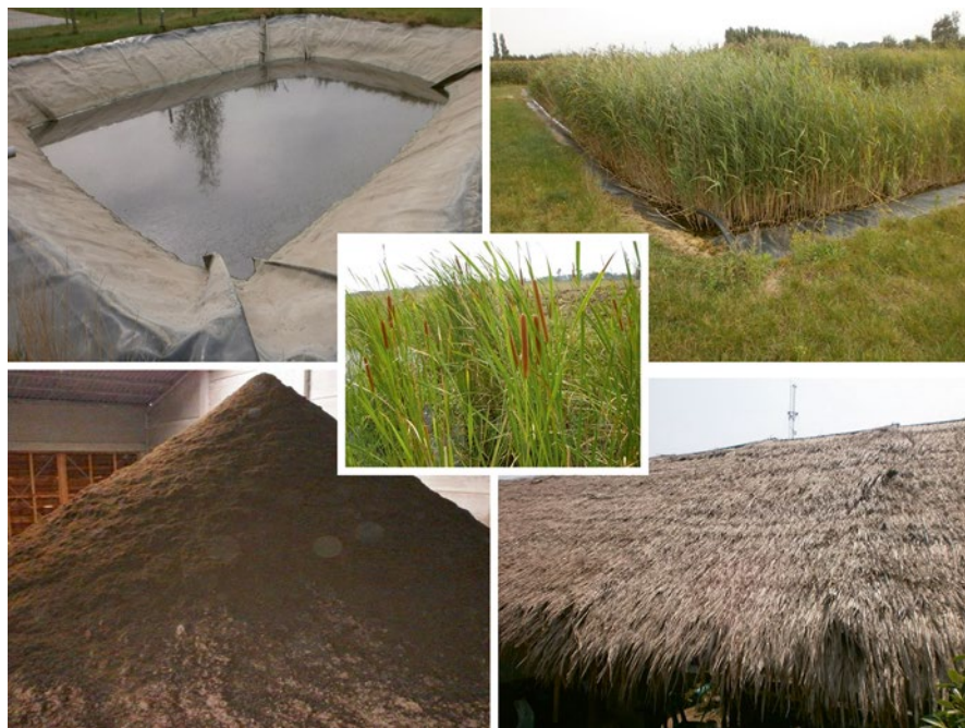
Fig. 7.52 Nutrient rich and sewage water treatment in constructed engineered wetland using high biomass produced macrophytes viz. Typha and Phragmites . Production of low cost roofing material and compost from macrophytes used in nutrient rich and sewage water treatment in constructed engineered wetland (Zhang et al. 2014; Zheng et al. 2013)
