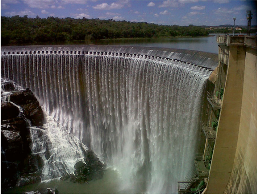
Fig. 4.2 Roodeplaat dam wall water spillage. This is the dam wall where water passes to various irrigation dams used for the supply of water for crop cultivation in the surrounding farmlands. Here, the water from the sewage water treatment plant at Zeekoegat that usually undergoes partial treatment mixes with another effluent water and water from other channels, which all together flows to the stream until it branches to the various irrigation dam in Roodeplaat farmlands. The dam used to be mainly for irrigation purpose until recently when it also serves as resort for recreation activities
