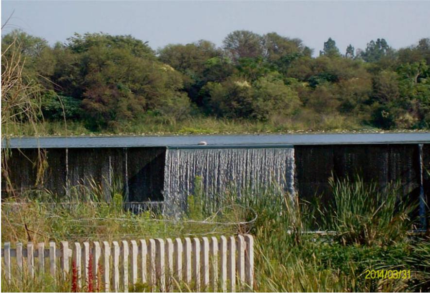
Fig. 4.1 High nitrate content water from Zeekoegat waste water treatment plant. The water is directly from the waste treatment plant, where solid waste from human are separated from sewage water. This water flows directly to the Roodeplaat Dam, where the water used for irrigation activities are sourced. Zeekoegat is a farming environment situated at the Northern part of Pretoria metropolis, South Africa. One of the Pretoria Municipality sewage water treatment plants is situated at Zeekoegat. This water is considered highly unsafe for drinking
