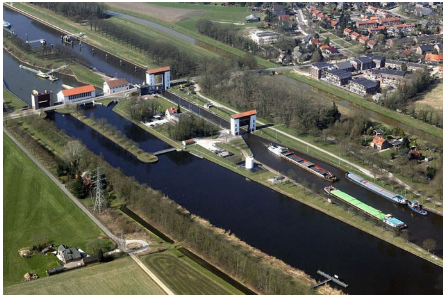
Fig. 5.1 All the structures of Lock Eefde, seen from the air. The lock itself is on the right . The two buildings on the left contain the discharge gates. The first white building from the left is the pumping station
