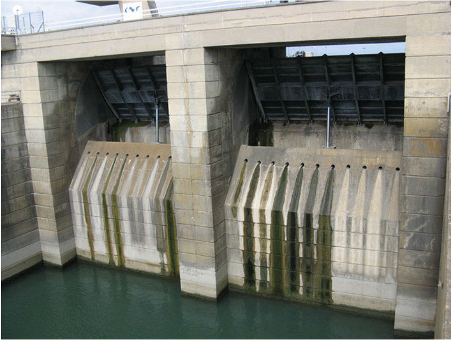
Fig. 3.4 Dam gates on the Rhône river—Vallabrègues plant
