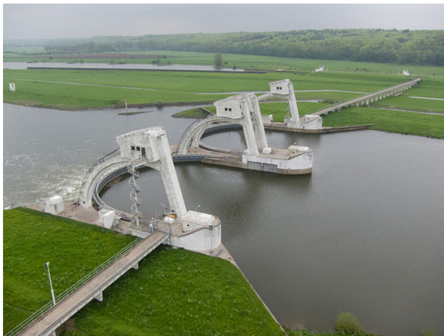
Fig. 11.3 The gate constructed at Driel for drought management (source: flickr.com\jasja_dekker)
