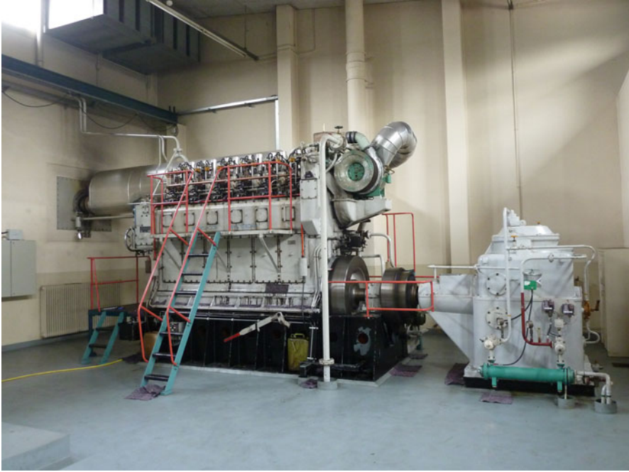
Fig. 5.12 One of the gasoline pumps at Lock Eefde, with a capacity of 5.5 \text{ m}^3/\text{s}
